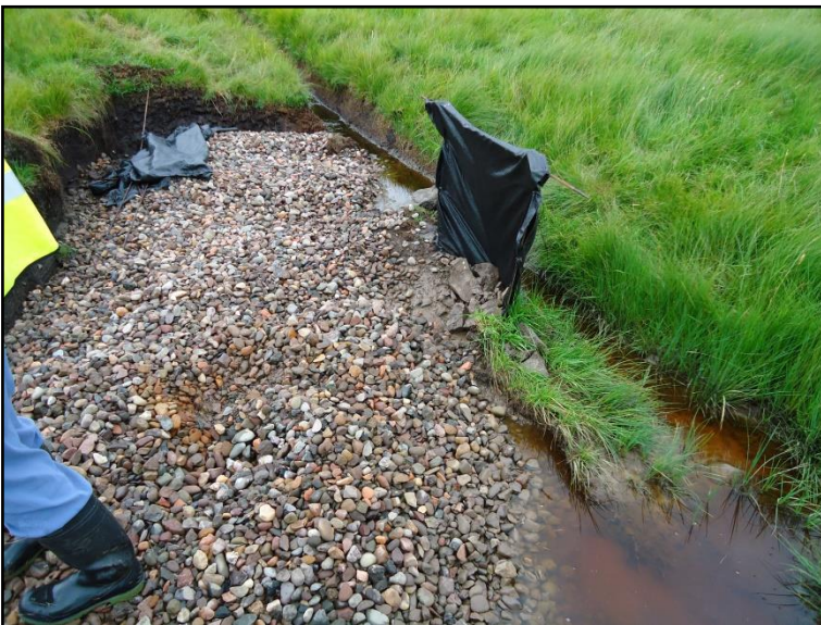
Plate 2: Typical silt traps
