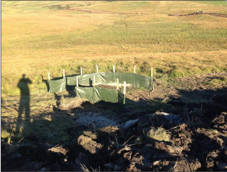
Plate 1: Typical silt fencing
